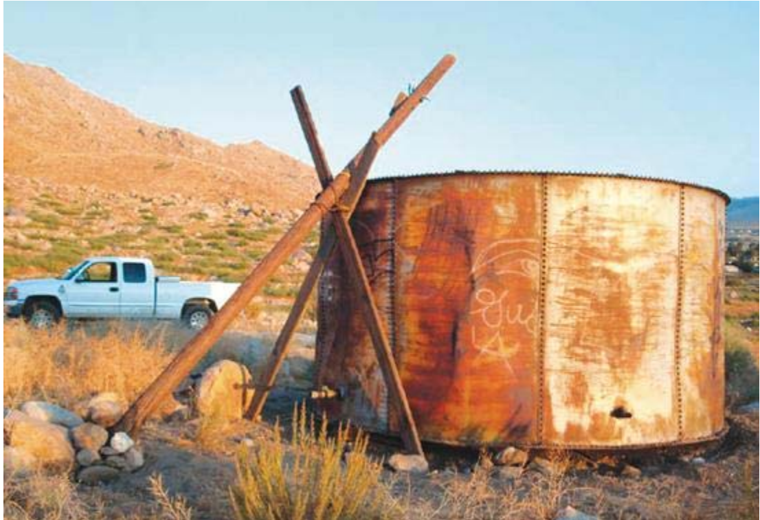
Would-be thieves built this wooden "A" frame hoist to lift this 3,000-pound water tank at the Cabazon Water District in an effort to take it apart to sell for scrap.
